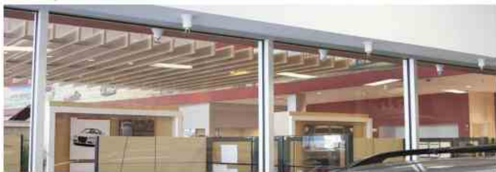
Window sprinklers used with glass partitions provide design choices that architects can use to create better building designs.
