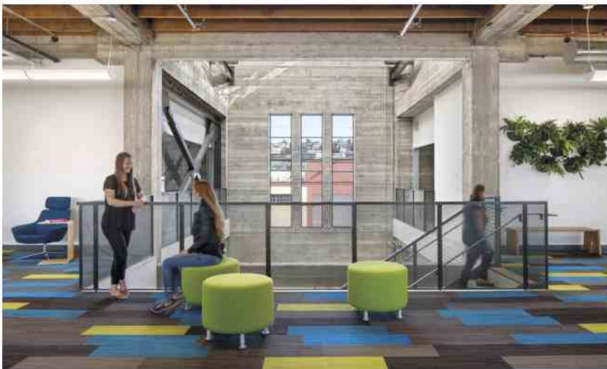
GOOD BONES Original wood roof sheathing, removed to create the atrium, now clads this space's walls (above). The two-story office building was opened up to pay homage to the adjacent warehouse, with exposed wood roof decking and both board-formed and existing concrete elements (left and opposite).
