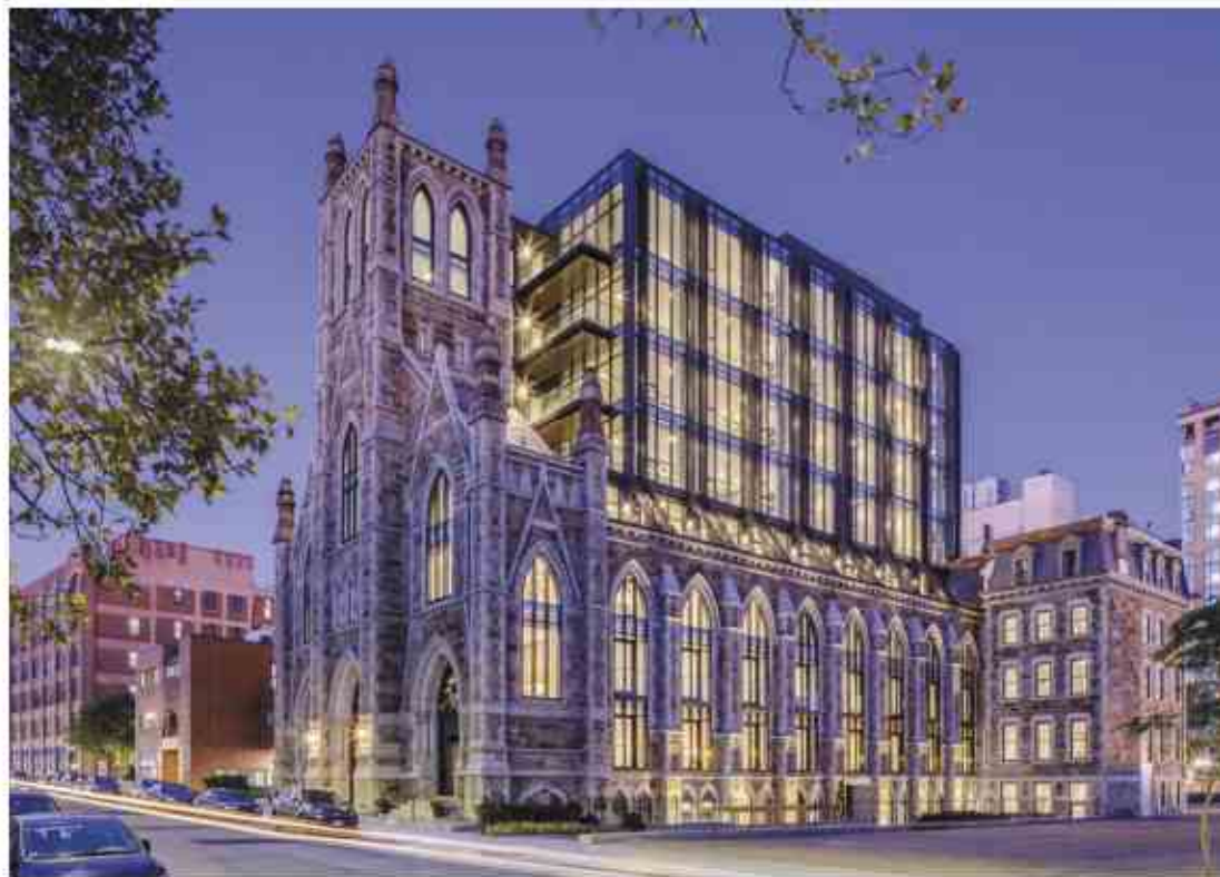
At Lucas, eight stories of condos have been inserted into the Gothic shell of the former German Trinity Catholic Church. Four floors of glass-and-steel-enclosed apartments rise above the late 19th-century building's old roofline, with new perimeter columns reading as an upward extension of the church's original stone structure.
