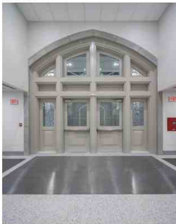
Custom-engineered blast-resistant doors were installed in a new barracks facility at the United States West Point Military Academy.
