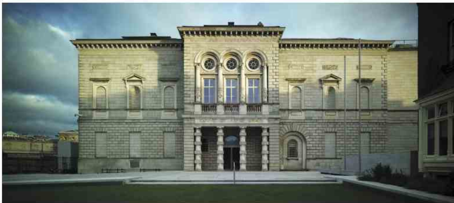
BACK TO THE FUTURE A new Wicklow granite ramp leads up to the main entrance of the historic museum; the team buried a mechanical space beneath the front lawn (above). Light bounces off original white-glazed bricks (opposite), illuminating the new minimalist courtyard around which visitors to the Dargan and Milltown wings now orient themselves.
