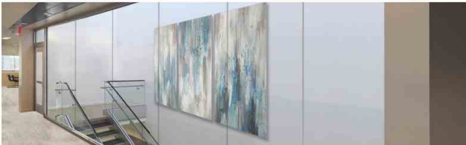
This 2-hour stairwell includes fire-resistive clear butt-glazed walls.
